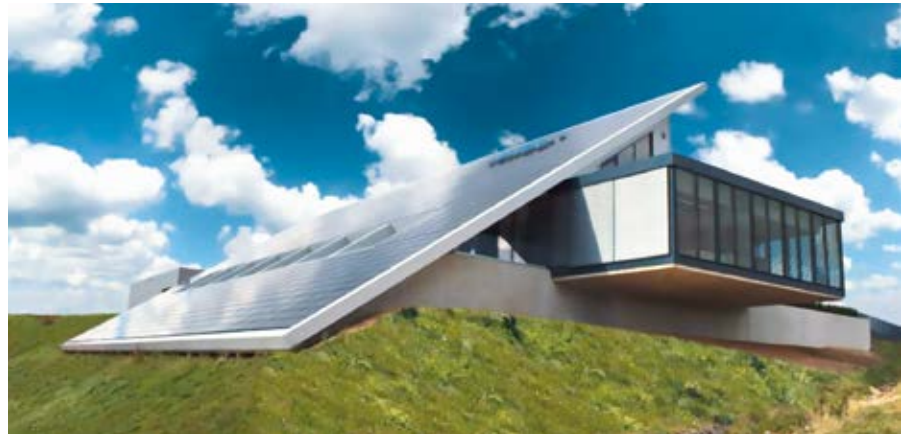
Modern building producing energy with CIGS solar modules (Modules provided by Avancis/CNBM)
